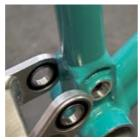
**FRAME ASSEMBLY** Place the black washer over the main pivot pin as shown and thread the male button head on. Cinch the button head down with a 5mm allen key while holding the opposing side with the 6mm allen key.
